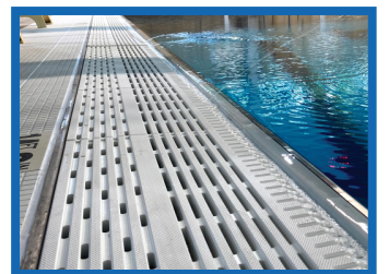
DECK DRAIN & PERIMETER GUTTER
